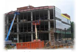
Fig. 4 - 6/29/07: Curtainwall grid installation on south elevation
